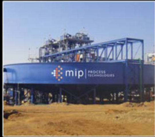
26m \phi Thickener in operation
